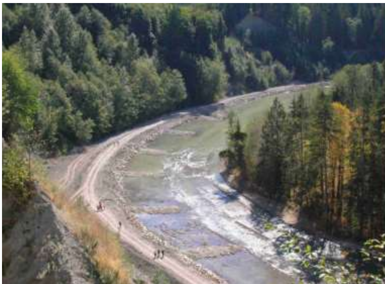
Photo 2. Downstream view of a series of 11 bendaway weirs constructed to train the thalweg away from the left bank along the Stoltz Slide in order to minimize bank erosion and the contribution of fine sediments (date and ref?)
